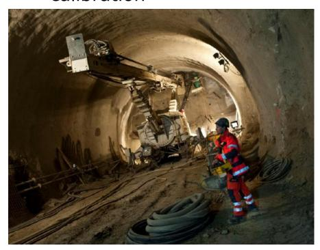
Tunnel face with relief drillings, before start of jet grouting works
